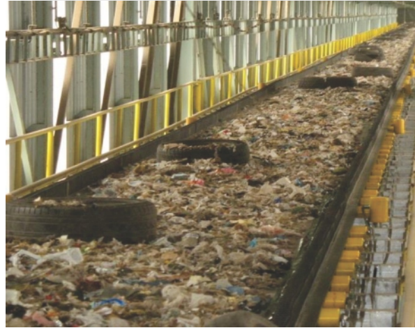
Fig: RDF & waste tyre handling system
