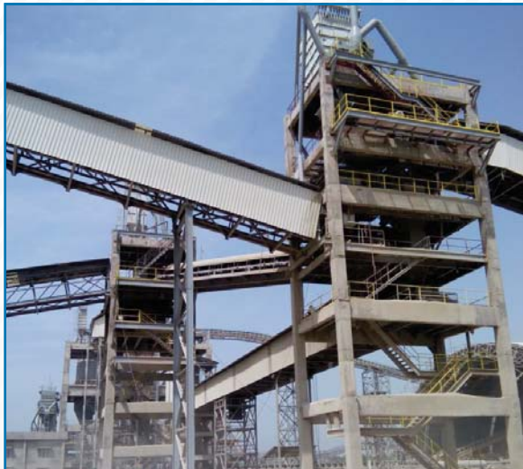
Limestone & Clinker Handling System at Reliance Cement
