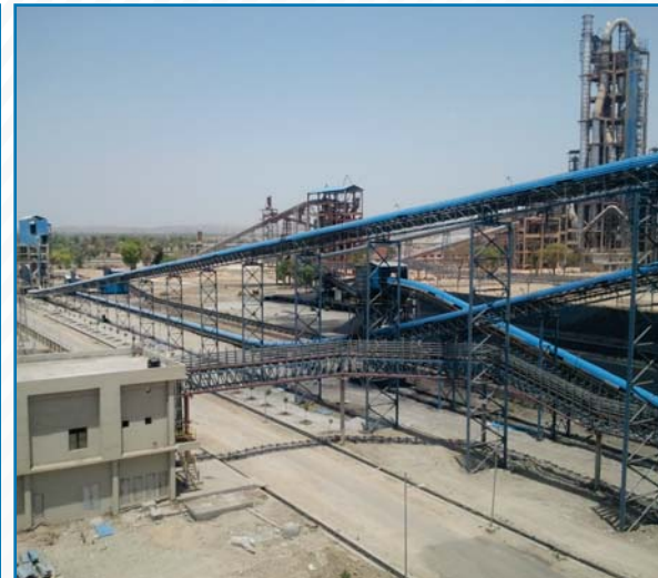
Coal & Limestone Handling System at Wonder Cement
