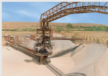
CIRCULAR STACKER RECLAIMER
